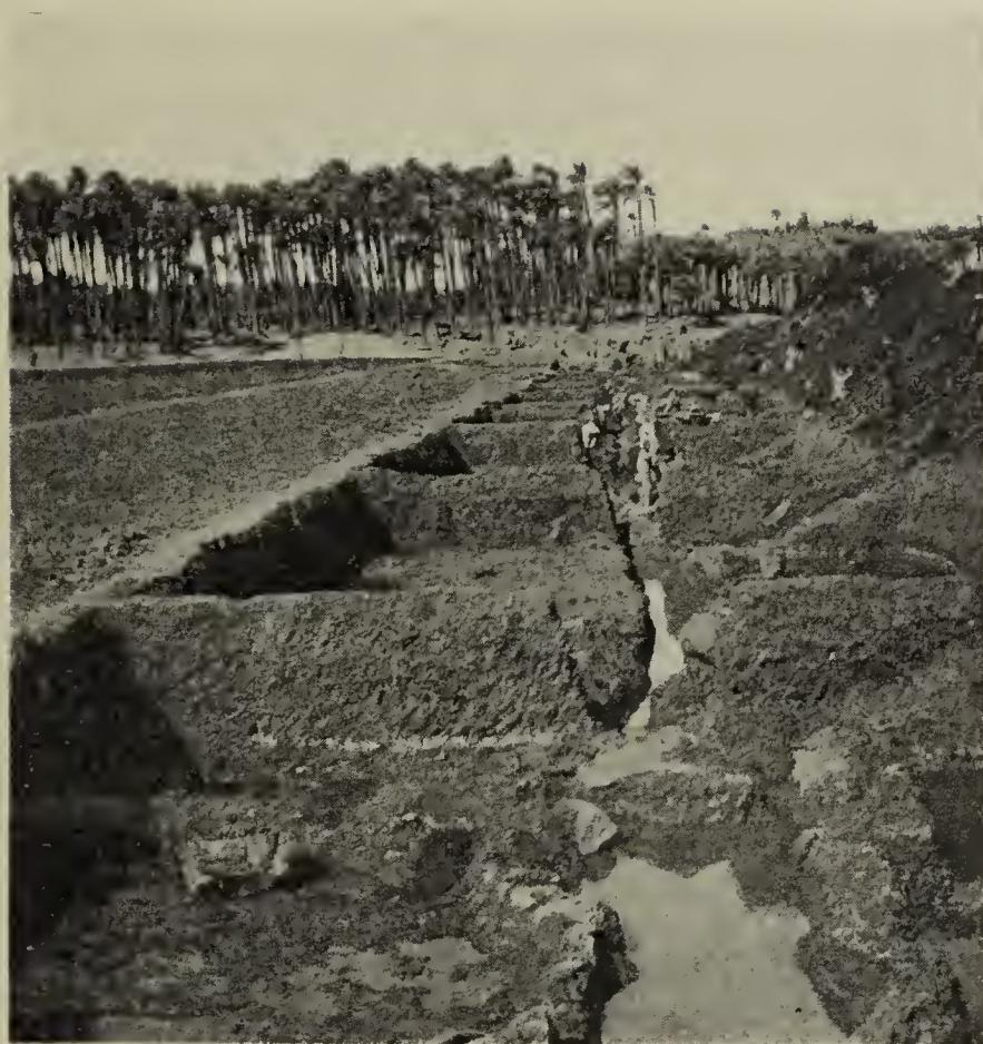
CANAL TO CARRY OFF THE WATER IN THE EXCAVATIONS
